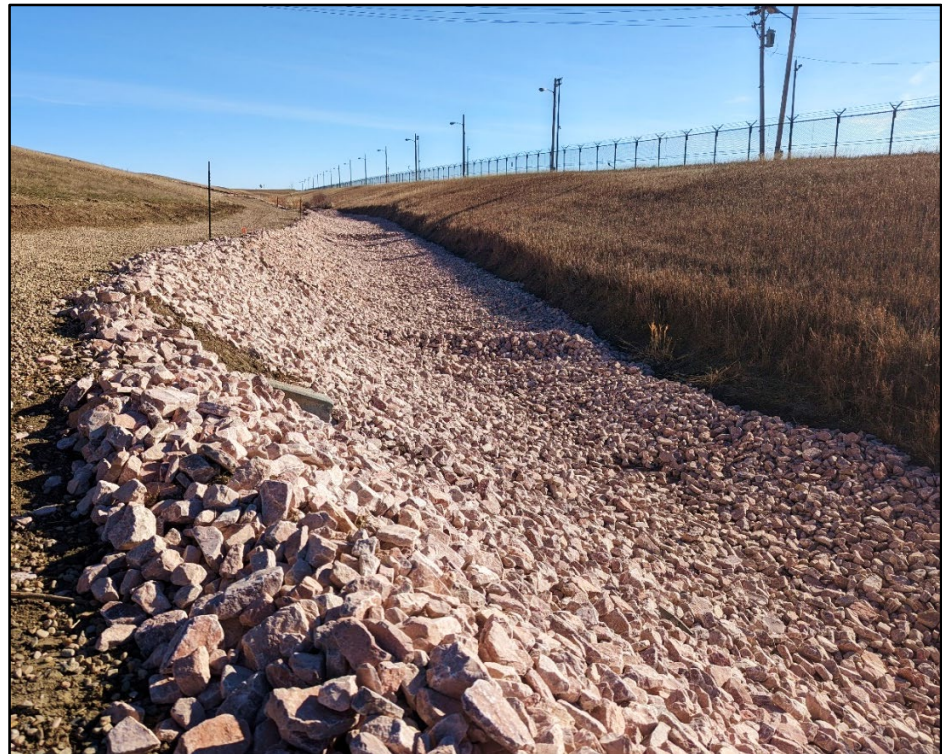
The surface water drainage after installation of the clay mats
