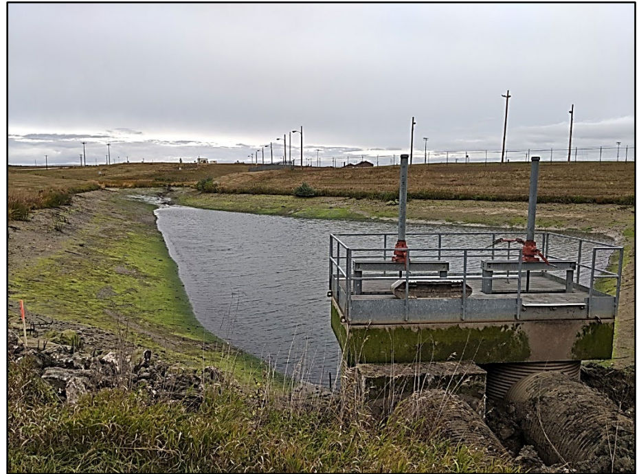
Pond 1, located directly south of the current and former fire training areas
