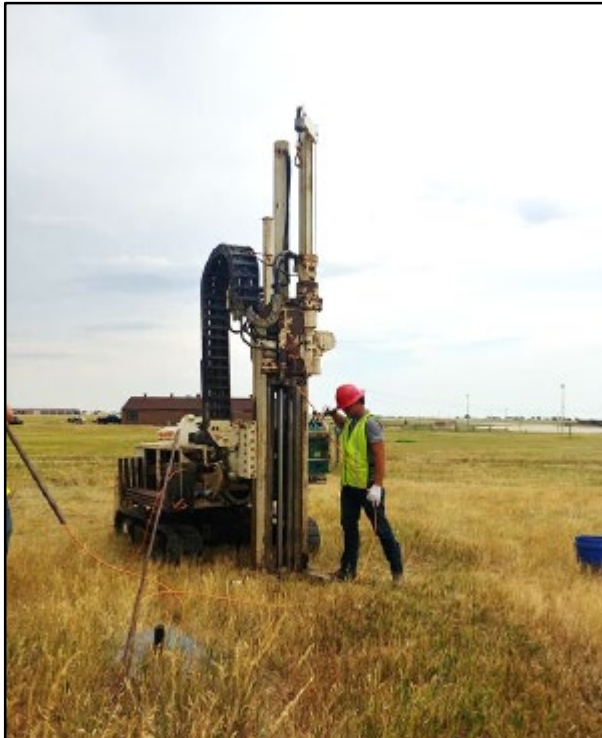
Drilling activities at the former fire training area prior to lysimeter installation
