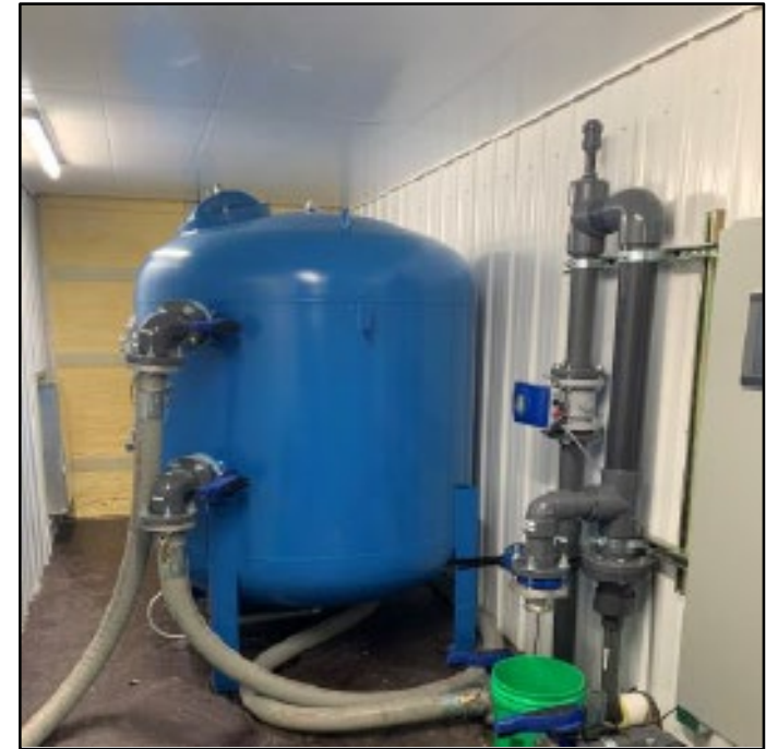
Ion exchange resin treatment vessel
