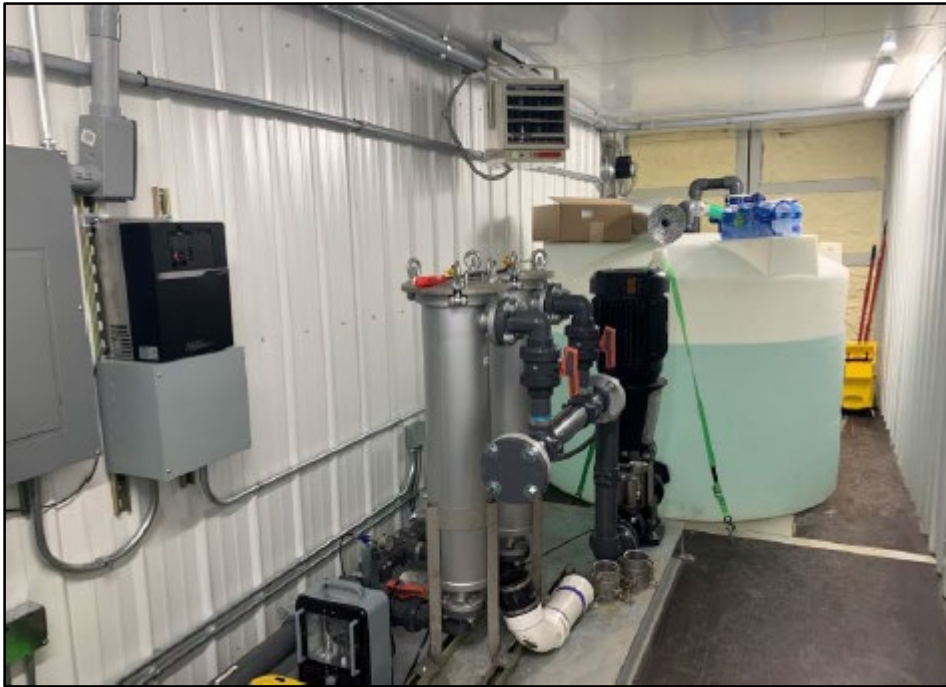
Bag filter assembly and equilibration tank
